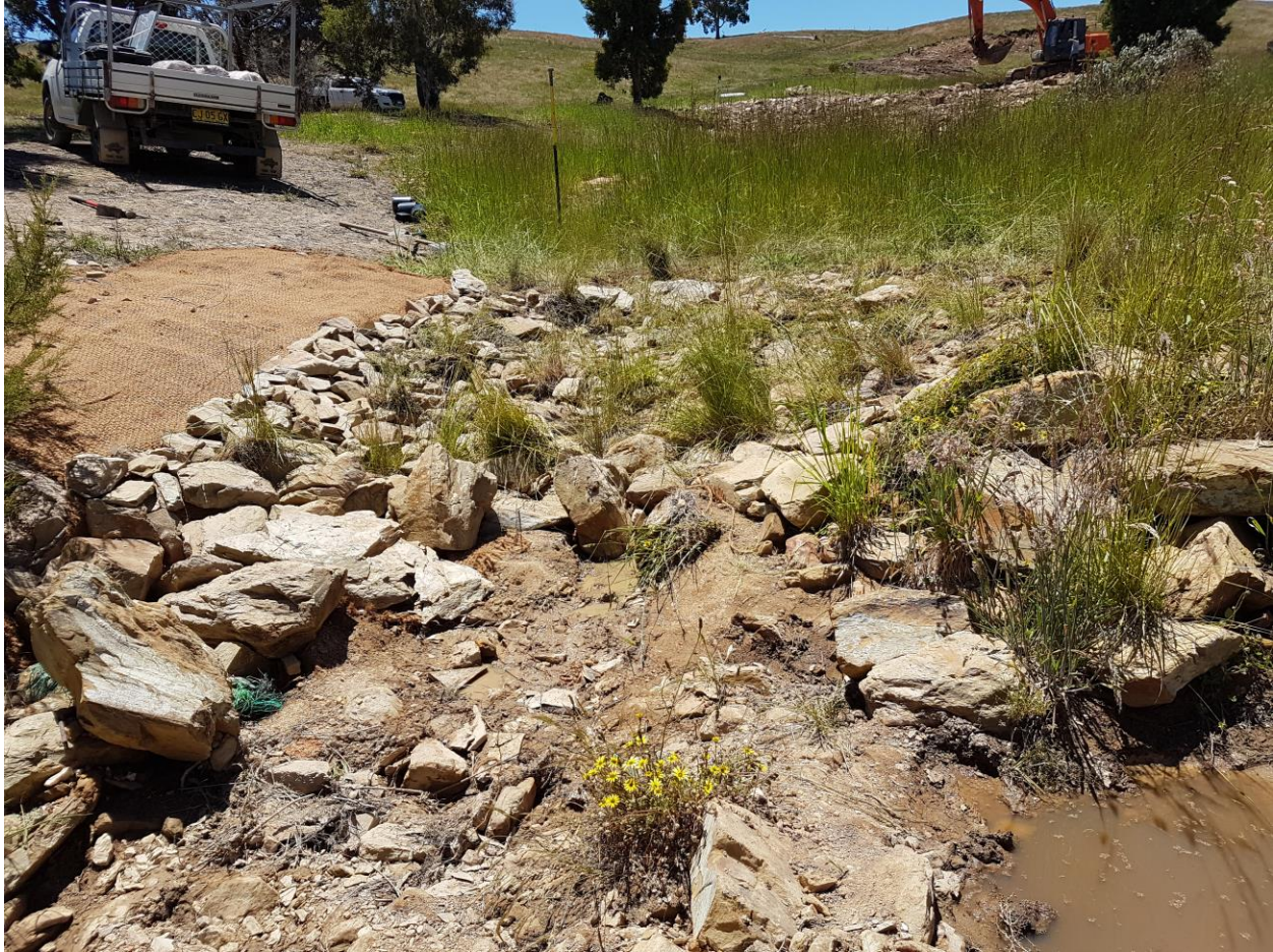
Figure 15. A rock flume was constructed to stabilise a headcut.
