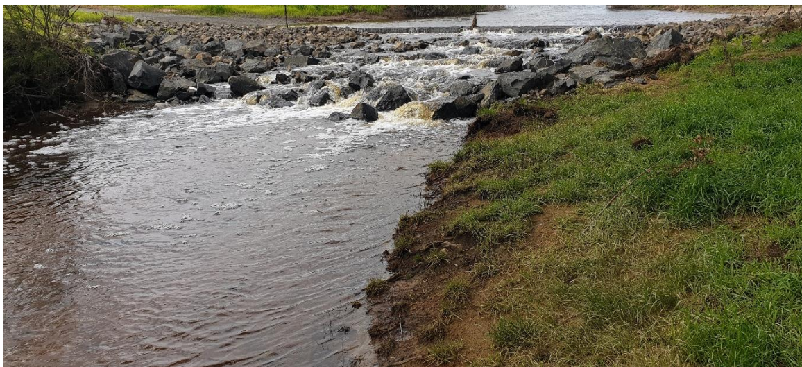
Figure 22. Completed leaky weir and crossing on Mulloon Creek at “Duralla”, March 2020.
